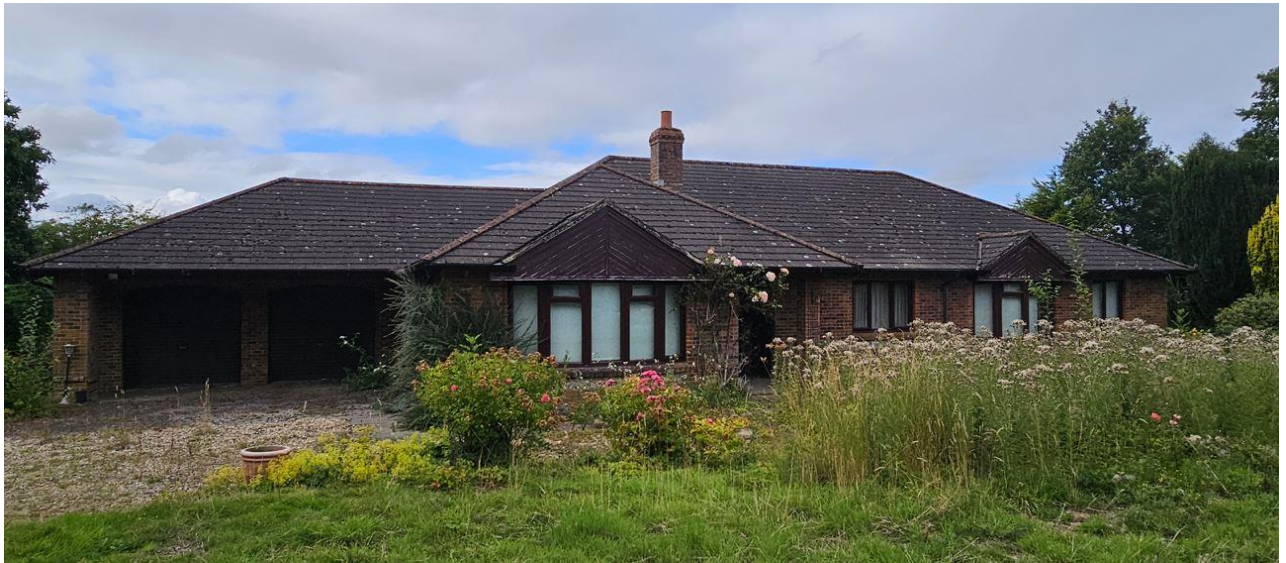
Figure 3 Front Elevation Photo
